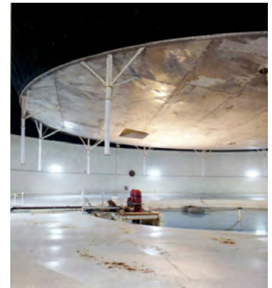
The "south lung" is one of the two rooms that allowed Biosphere 2 to breathe—and not explode—during its former life as a closed structure.
